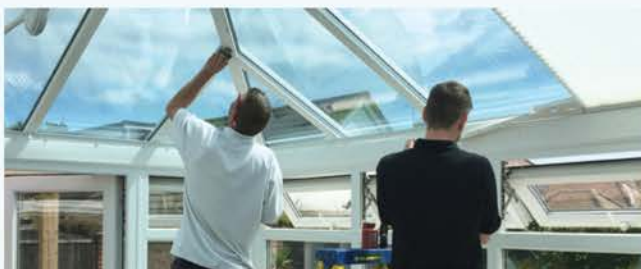
Installation is carried out by our experienced fitters
